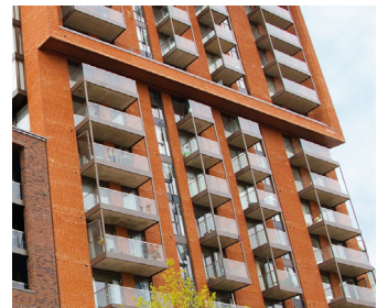
Photo: Sapphire Balconies
