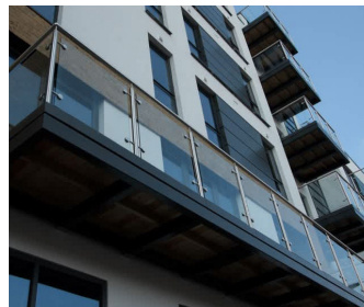
Photo: Sapphire Balconies
