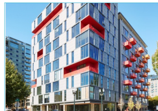
Use of colour, modest facade modulation, use of recessed and extended balconies.
