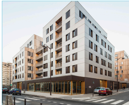
Lower overall WWR with an active, transparent frontage.
