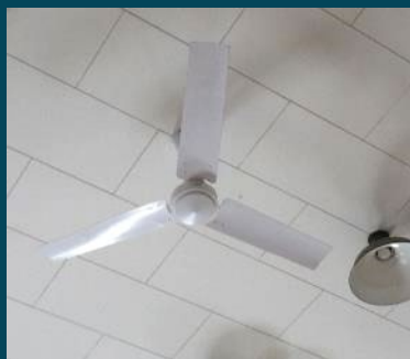
Figure 4.5: Examples of mechanical systems that provide limited cooling demand reduction: ceiling fans (left), exhaust fans (middle), and continuous exhaust/heat recovery ventilators (right).
