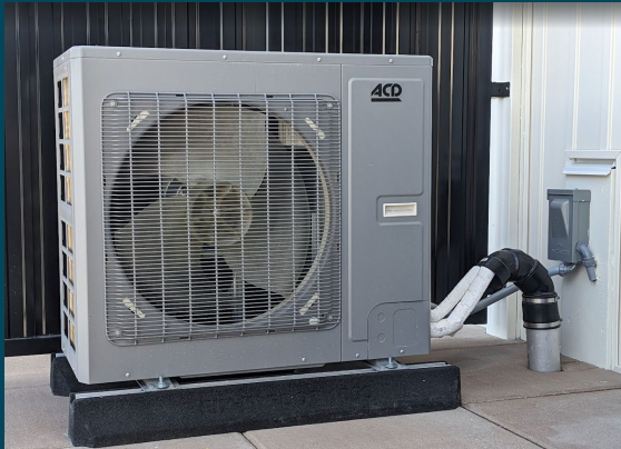
Figure 1.1: Example mini split heat pump condenser placement for a Part 9 single family home (left) and a low-rise Part 3 multi-unit residential building (right).
