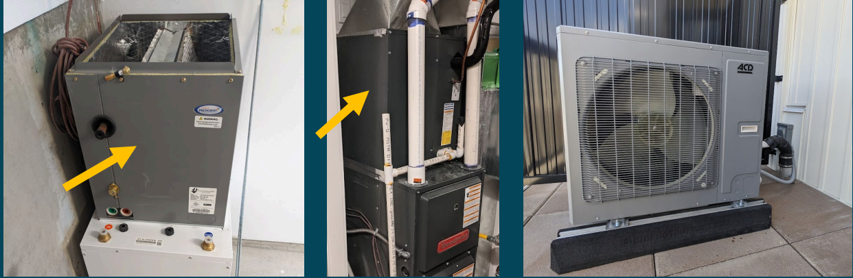
Figure 5.2: Examples of heat pump system components: indoor heat exchangers in central forced-air systems (left and middle) and outdoor air-source heat pump unit (right)
