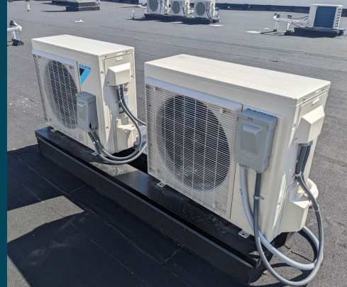
Figure 1.1: Example mini split heat pump condenser placement for a Part 9 single family home (left) and a low-rise Part 3 multi-unit residential building (right).
