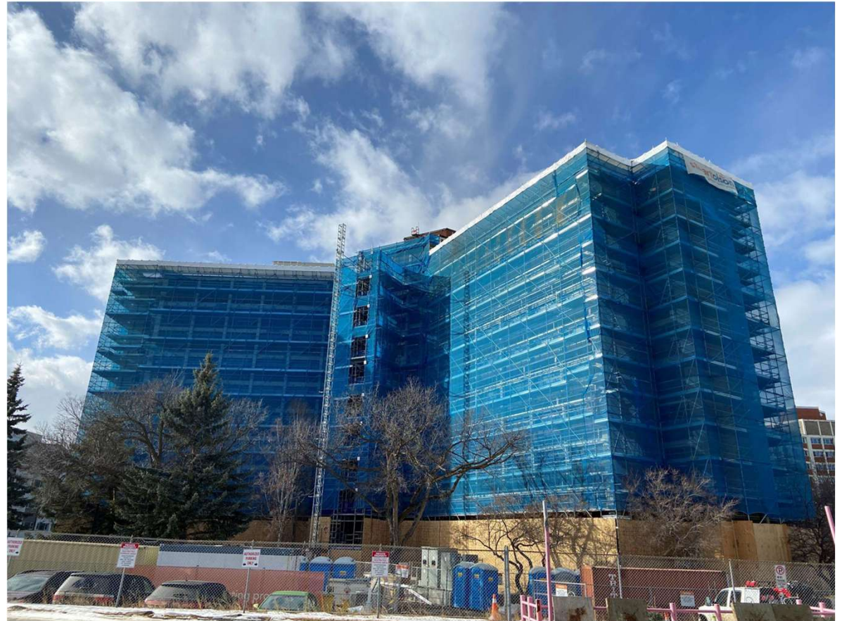
MACKENZIE HALL – 1 of 3 BUILDINGS
