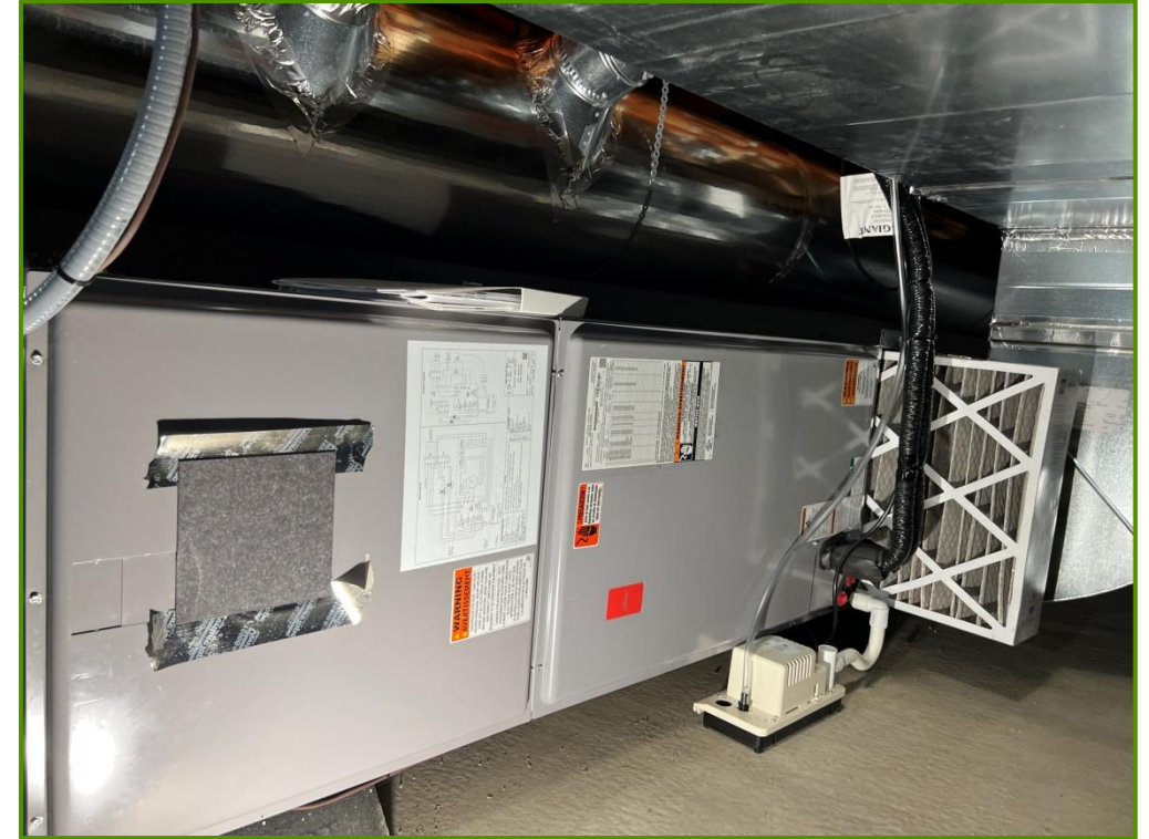
Accessible filter cabinet with 5" pleated high-efficiency filter
