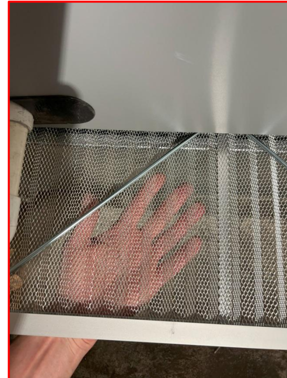
Metal screen “filter” installed
