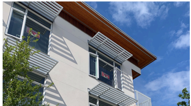
Example of the use of exterior shading devices to limit solar gain and overheating potential (The Clive, Victoria BC).
