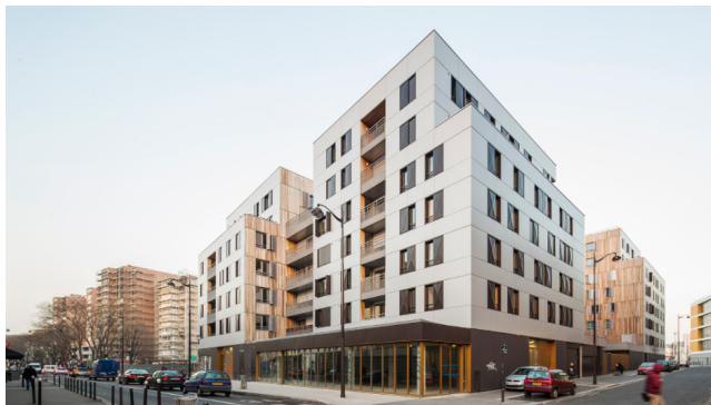
Example of a building with an active frontage and low overall WWR.
